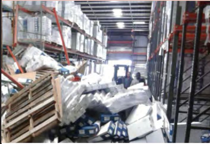
The incident shown above could have been avoided. This collapse was caused by a lack of consistent warehouse rack inspections. Failure to address damaged and missing pallet rack components led to this tragedy. Fortunately, no one was injured in the scenario but it could have been prevented by regular warehouse rack inspections and repair or replacement of damaged pallet rack components.
